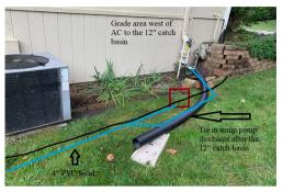
2: Before the trenching starts, utility locates will be called in by Lawrence Landscape. After the trench is dug, a clean gravel base is installed to act as a bed for the perforated pvc pipe with a silt filter sock to rest on.
