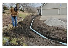
Once the pipe is installed, a clean washed gravel will be added until the pipe is covered. For the best performance, a Decorative River Gravel is placed on top, The traditional French drain will have soil added back and sod installed.
